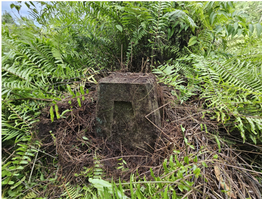
Concrete pillar base of the Highland Lumber sawmill in San Juan.
